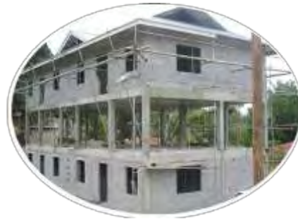
Commercial Building under construction
